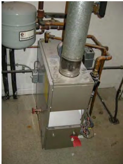
Typical gas-fired boiler
