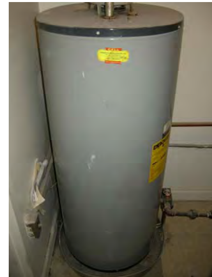
Typical gas-fired storage water heater
